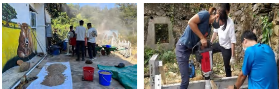
Fig.17. Soil preparation. Fig.18. Ramming.
